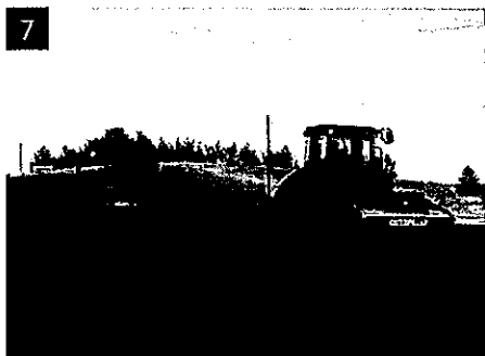
7 Vibratory pad-foot compactor followed by the pneumatic version to achieve a smooth top surface
