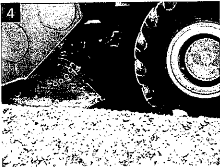
4 A second pass with the reclaimer to blend TerraCem into the soil
