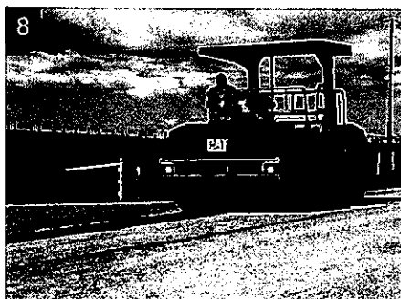
8 Smooth drum compactor for the final finish of the subgrade
